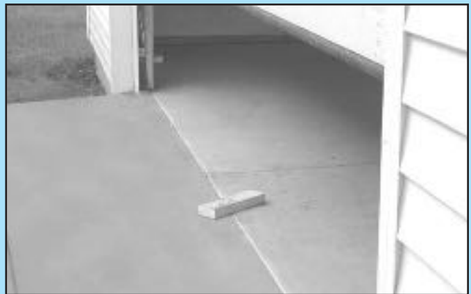
FIG. 6-5 2 x 4 under center of door opening.
